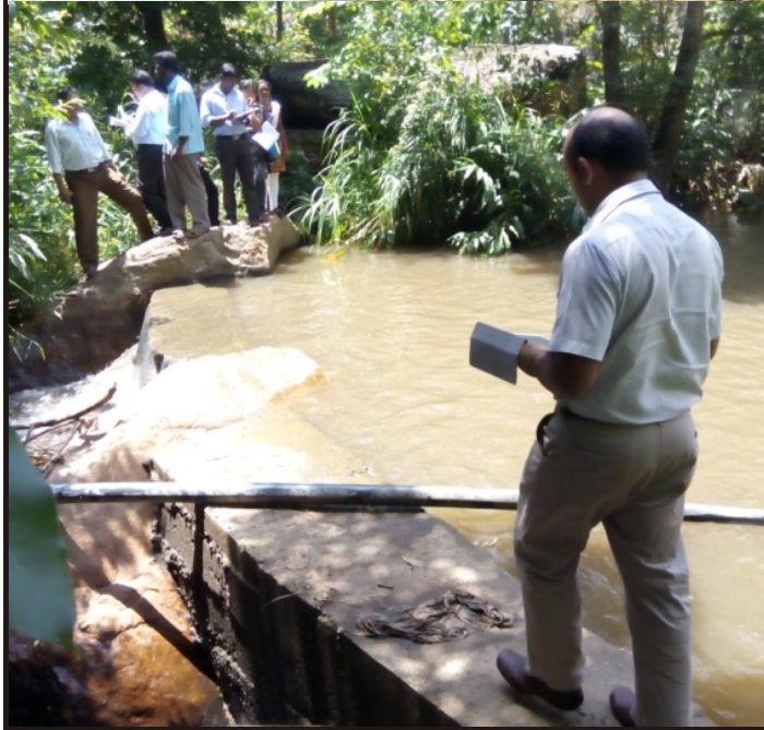
Source Development Check dam @ Thpputhura
